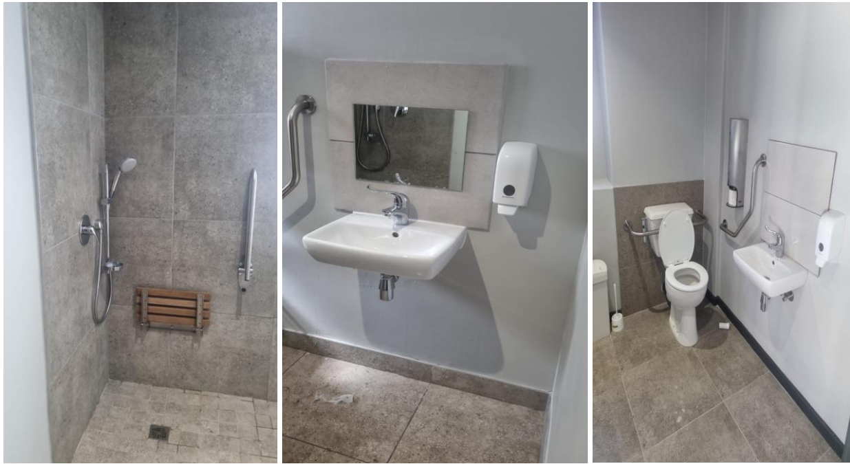
Figure 17: Bathroom for persons with disabilities
